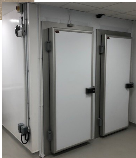
-30°C freezer system and 3°C Fridge installation
